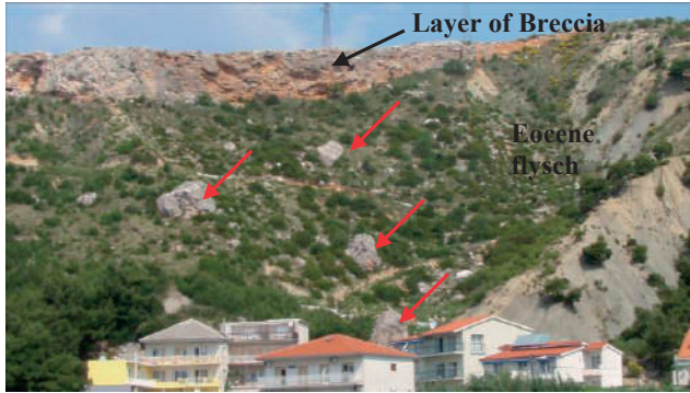
Figure 3 South-east view of the rock cliff at Luka location. Slope is made of Eocene flysch with layer of breccia marked by black arrow. Larger detached blocks are marked with red arrows.
