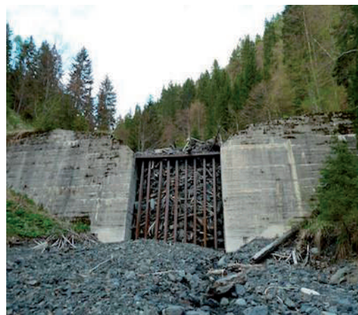
Figure 9 Example of a filled concrete check dam in the Suhelj Torrent with a filtering function.
