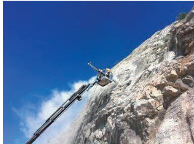
Figure 6 Installation of geotechnical selfdrilled rockbolts on high steep slopes.
