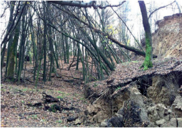
Figure 3 One of many secondary tension cracks at landslide 2.
