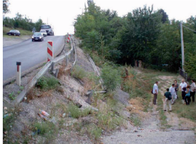
Figure 3 Deformation on the road M-19.
