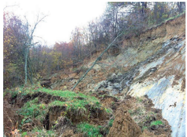
Figure 2 Main scarp of landslide 2 in the Torine Quarry.
