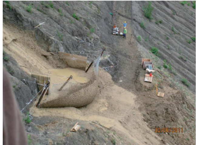
Figure 5 Completely with mud filled test barrier in Veltheim.
