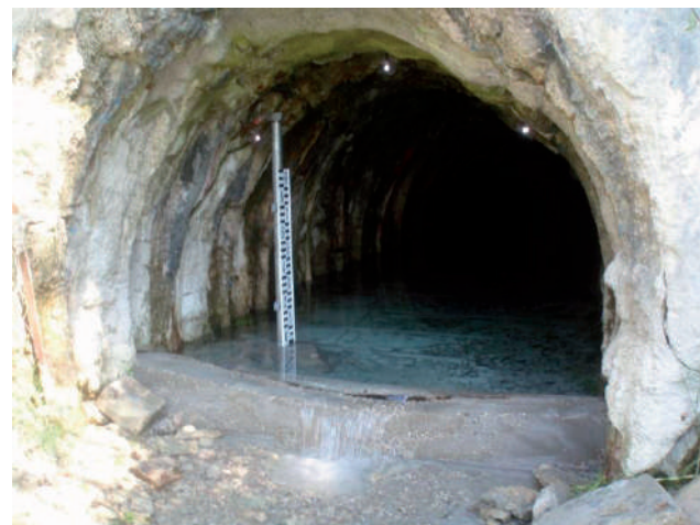
Figure 5 Entrance of the tunnel with outflow weir.
