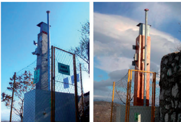
Figure 4 Concrete main pillar housing for robotic total station on the top at the Veli Vrh location before insulation is applied (left) and after thermal insulation is applied (right).
