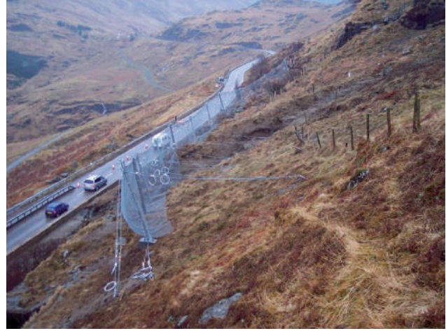
Figure 9 Installed landslide barrier.
