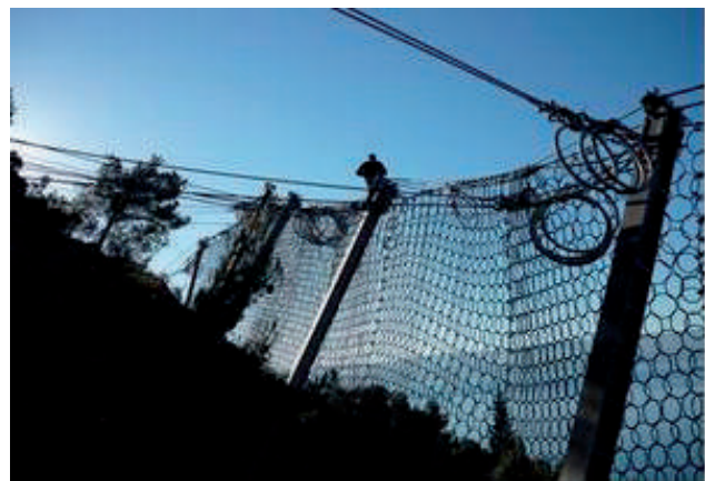
Figure 7 Installation of high energy absorption rockfall protection barriers.
