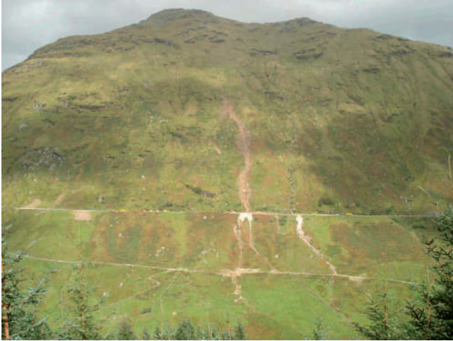
Figure 2 Shallow landslide events at Rest and be Thankful along the slope 2009 (picture source Scotland Transport).
