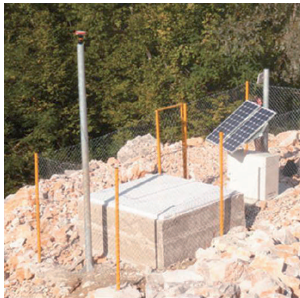
Figure 3 GPS rover and prism at the top of the pole and solar panel installation at the control point B3 in the Grohovo Landslide. Concrete box is round up construction for geotechnical monitoring equipment protection with inclinometer casing, vertical extensometers and pore pressure gauges inside (Arbanas et al. 2012a).
