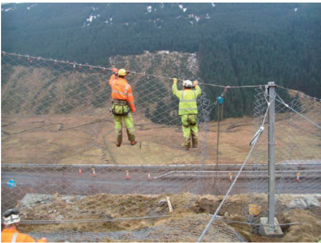
Figure 8 Installation of Landslide barrier.
