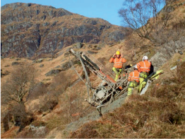
Figure 7 Drilling for the anchors.
