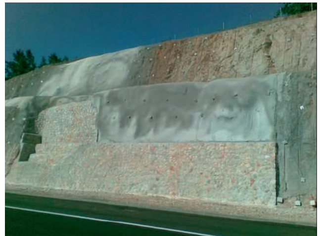
Figure 4 Rockfall protection using reinforced shotcrete and stone lining.
