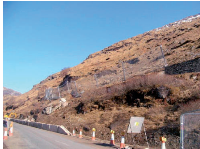
Figure 10 Landslide barrier near road.
