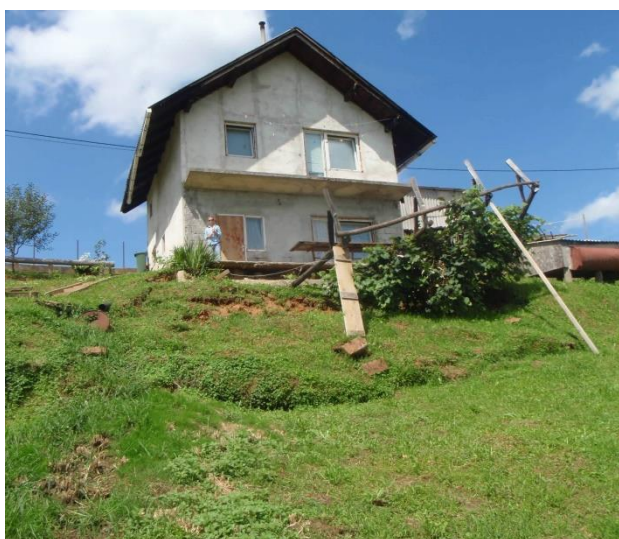
Figure 4 Example of a High Risk landslide.
