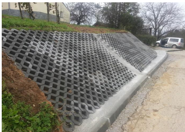
Figure 10 Landslide remediation with prefabricated concrete elements.
