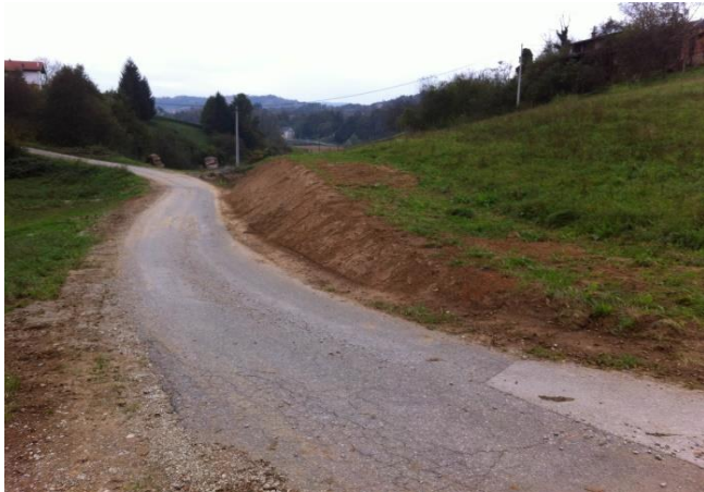
Figure 12 Low Risk landslide remediation by arrangement in stable slope.
