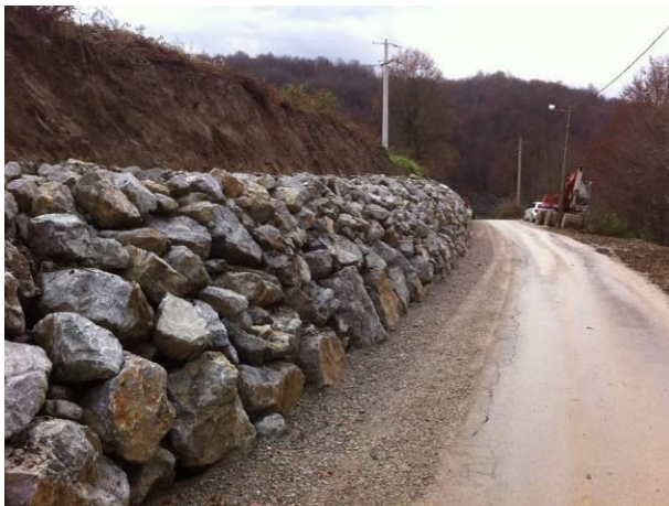
Figure 8 Landslide remediation with stone retaining wall.
