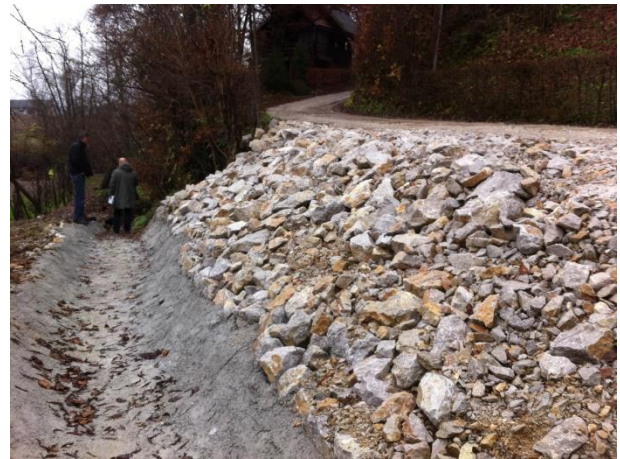
Figure 9 Landslide remediation with stone retaining wall.
