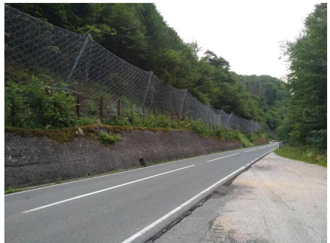
Figure 9 New net barrier installed above the older protection measures.
