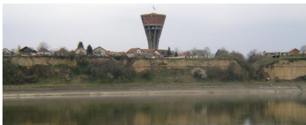
Figure 6 Along the right bank of the Danube river are regular occurrences of landslides and escarpments.
