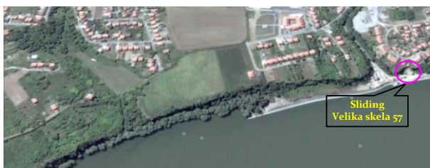
Figure 8 Landslide Velika Skela 57 activated in August 2008.
