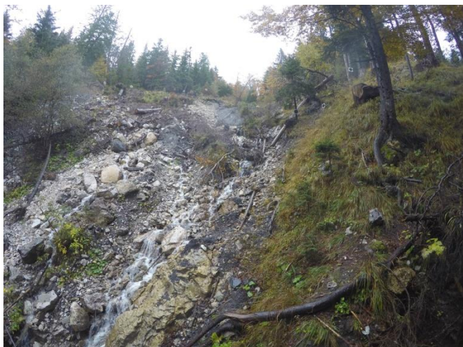
Figure 4 Sample landslide photo of landslide.
