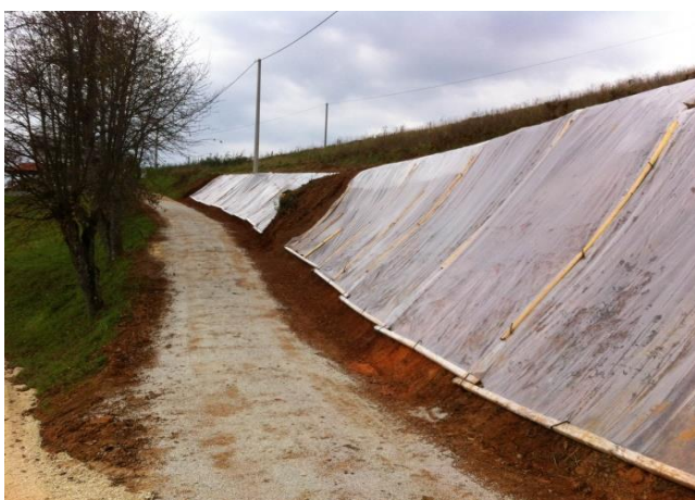
Figure 11 Temporary slope protection on a Low Risk landslide.
