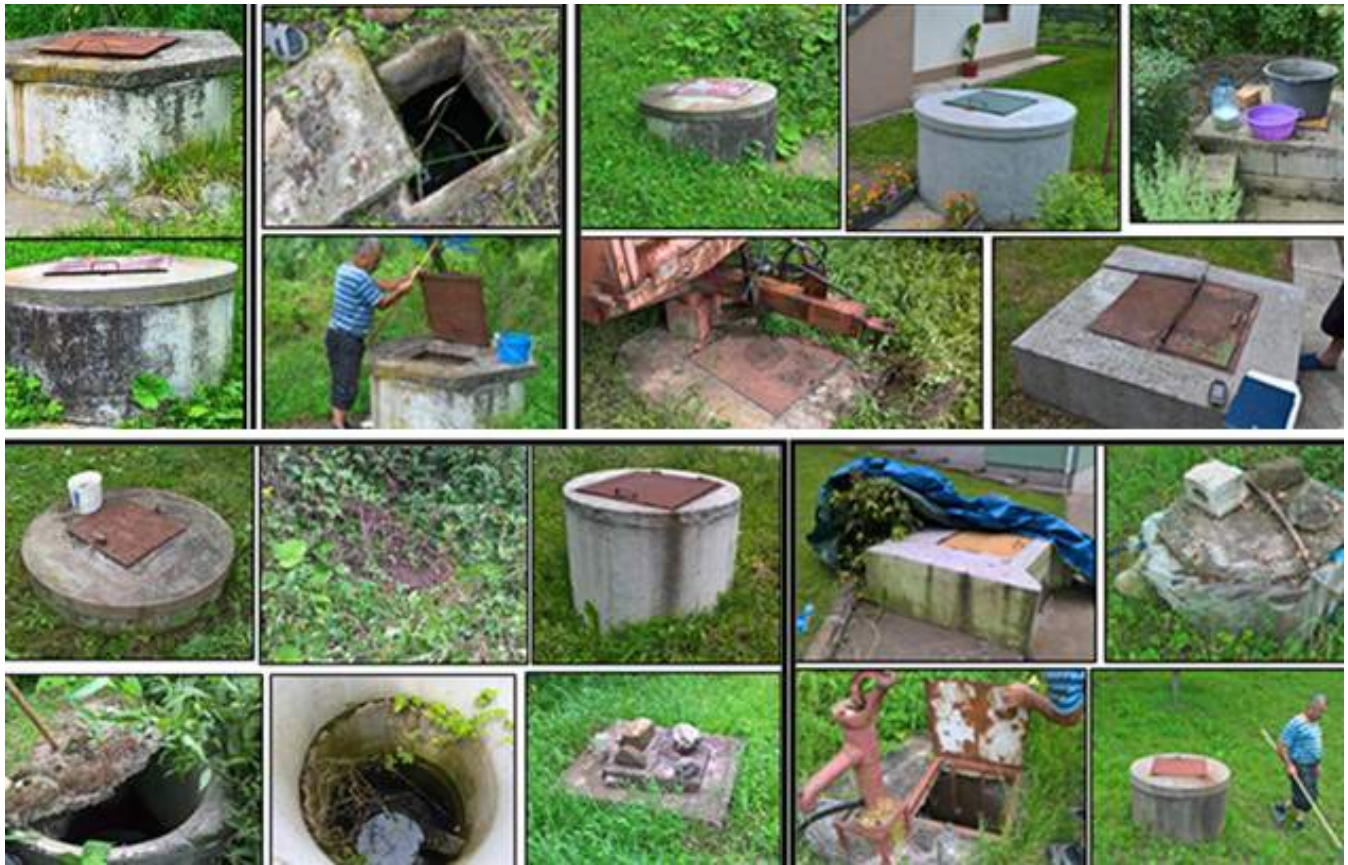
Figure 5 Registered dug wells on the landslide
