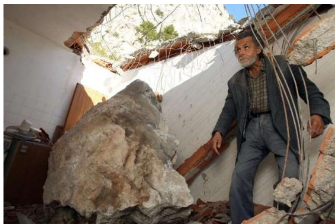
Figure 2 Fallen rock block came through the roof in the house in January 2012 ( www.24sata.hr ).
