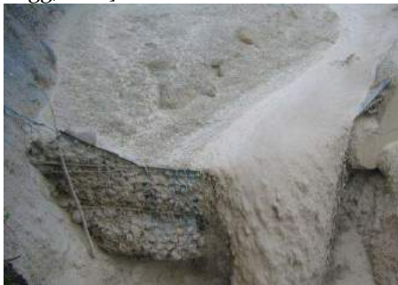
Figure 1 Flexible ring net barrier withstanding overflow in the Illgraben.
