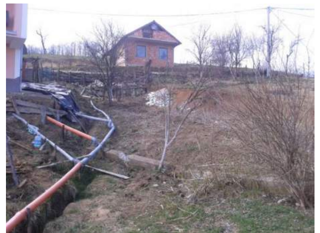
Figure 7 New plastic pipes instead of crumpled
