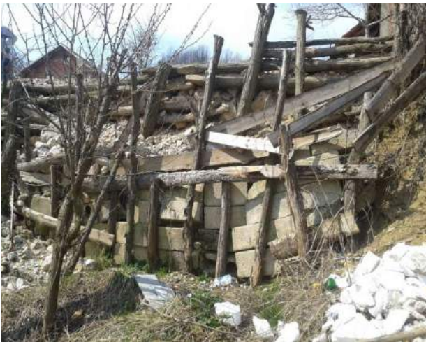
Figure 8 Temporary road repair
