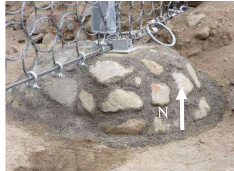
Figure 5 Scour protection around the posts for UX-barriers
