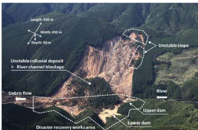
Figure 9 Landslide dam and unstable colluvial deposit (Sato et al. 2014)
