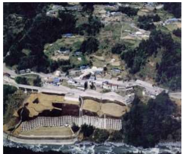
Figure 5 Landslides in metamorphic rock formation
