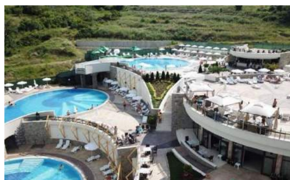
Photo 5 The landslide, the retaining wall and the aquapark
