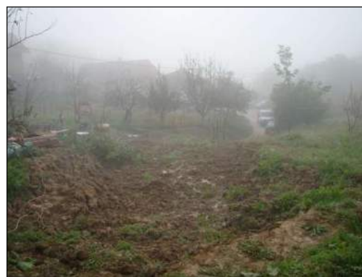
Figure 1 Landslide photo, a sliding mass that has been gravitationally moved along the road.
