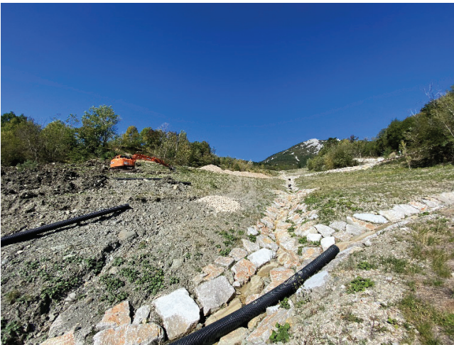
Figure 8 Excavating work on the landslide in October 2021.
