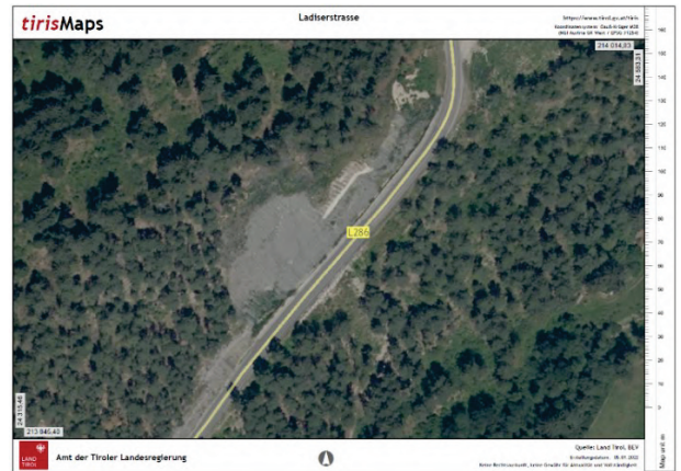
Figure 16 Orthophoto of the stabilised slope along the Ladiserstrasse (tirisMaps, 2018).
