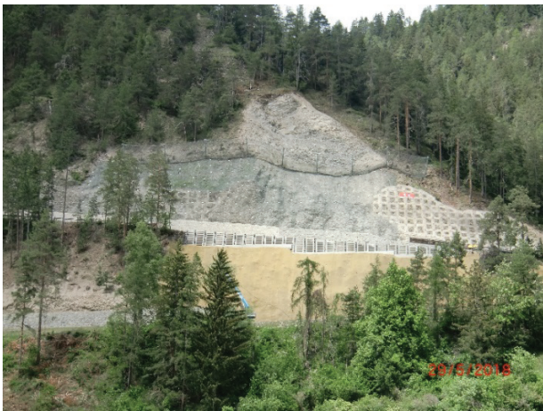
Figure 20 Serfauserstrasse stabilised slope, with a rockfall barrier at the top, anchored high-tensile steel mesh in the middle and greening mats in the bottom part of the slope.
