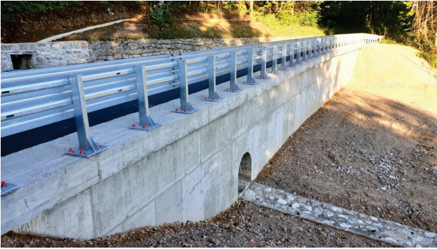
Figure 7 Dedin landslide on state road DC3 (section 015) at km 2+060 after remediation works.
