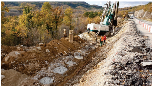
Figure 8 Remediation works on pile wall at Vranja landslide.
