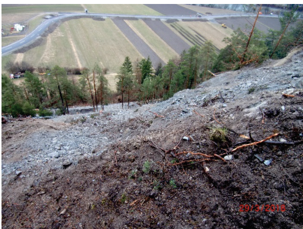
Figure 7 View from top of the landslide along the Serfauterstrasse, approximately one month after the event.
