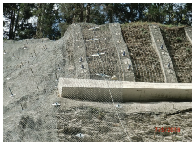
Figure 12 Stabilisation of the concrete ribs that were undamaged during the slope failure, with a concrete anchor beam and high-tensile steel mesh cover. Note the larger spike plates in this section, belonging to the TECCO system, which can support higher loads.
