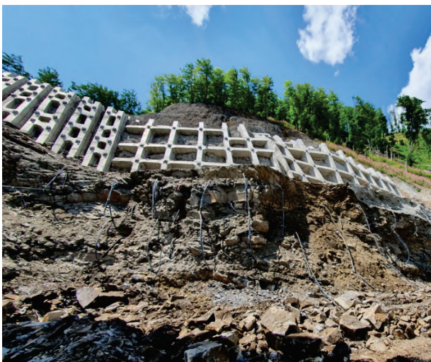
Figure 7 Photo of remediation measures.
