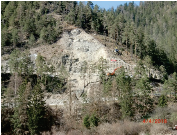
Figure 13 View of the unstable slopes along Serfauterstrasse.
