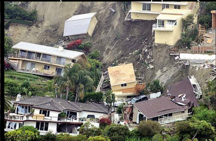
Laguna Beach landslide, California, 2005
